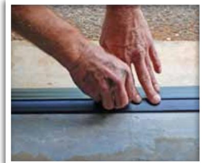
8. Close the garage door to keep constant pressure on the threshold for twenty-four (24) hours.
