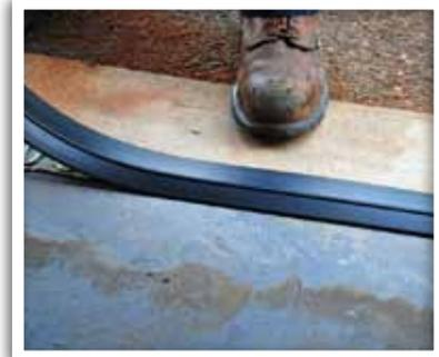
7. Inspect the threshold to make sure it is still between the pencil lines. The position can be slightly adjusted for a short period of time. The length of time varies depending on ambient conditions.
