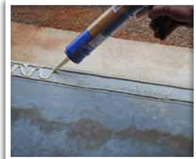
6. Replace the threshold between the pencil lines and firmly press into place. Carefully apply pressure to the threshold to ensure the adhesive spreads uniformly.
